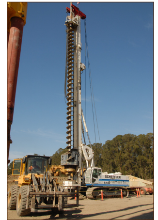
A drill can go 100 feet down into bedrock.
